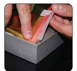
Insert narrow side of silicone welt into the channel at corner **1**, with fabric to the outside.
